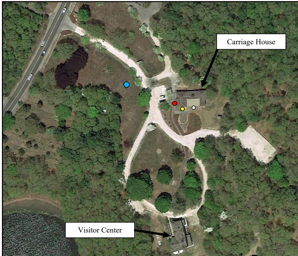
Figure 2: The image above shows the Waquoit Bay NERR Headquarters. The red circle marks the location of the current 30-foot tower location (November 2015 – present). The yellow circle marks the past location of the wind/temperature/relative humidity tower (2006 – August 2015). The white circle marks the location of the photosynthetically active radiation sensor prior to April 18 th , 2016, when the sensor was moved to the 30-foot tower (red dot). The larger blue circle indicates the location of the precipitation gauge in the open field. The barometric pressure sensor is located inside the Carriage House in the laboratory along with the CR1000 logger. Aerial provided by Google Earth (spring 2015).
