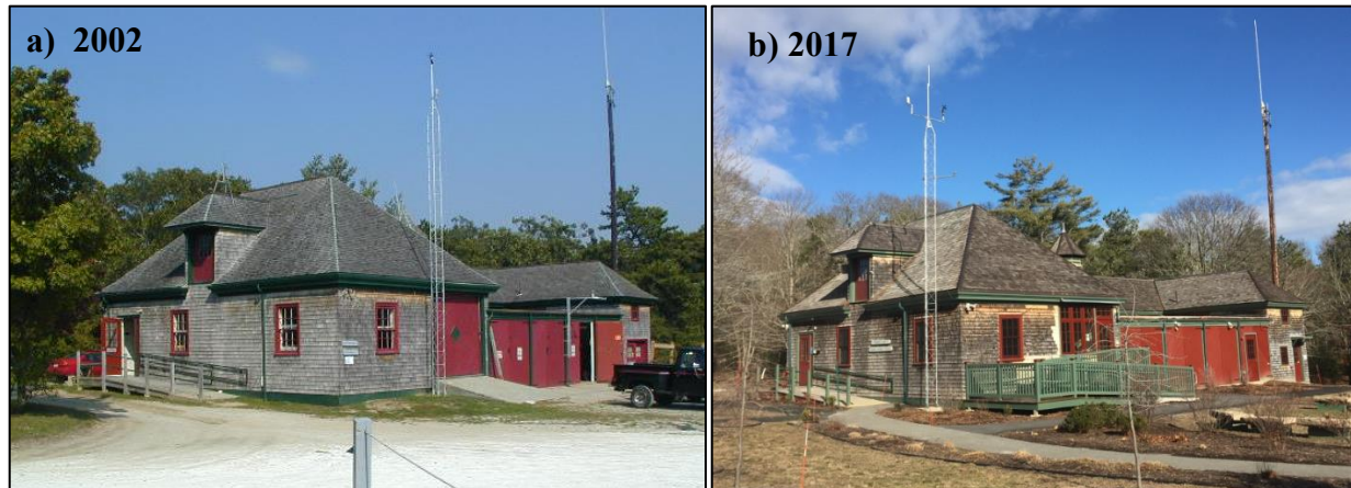
Figure 1: Photos of before (a) and after (b) the 2015 Carriage House renovation and the 2016 tower upgrade. The tower upgrade in 2016 involved a new lightening rod, grounding wire, cross bar, and upgraded temperature/relative humidity and photosynthetically active radiation sensors.
