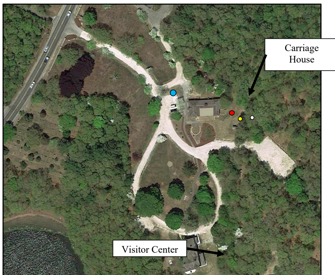
Figure 2: The image above shows the Waquoit Bay NERR Headquarters. The red circle marks the location of the current 30-foot tower location (November 2015 – present). The yellow circle marks the past location of the wind/temperature/relative humidity tower (2006 – August 2015). The white circle marks the location of the photosynthetically active radiation sensor prior to April 18 th , 2016, when the sensor was moved to the 30-foot tower (red dot). The larger blue circle indicates the location of the precipitation gauge in the open field. The barometric pressure sensor is located inside the Carriage House in the laboratory along with the CR1000 logger. Aerial provided by Google Earth (spring 2015).
